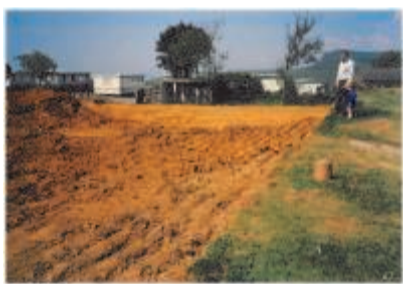
Swimming Pool Foundations
