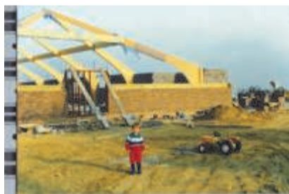
Swimming Pool Building
